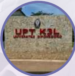
Integrated Waste Treatment Plant (IWTP)
