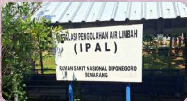
Wastewater Treatment System
