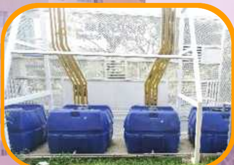
Element 5 Water Efficiency Water Harvesting & Recycling
