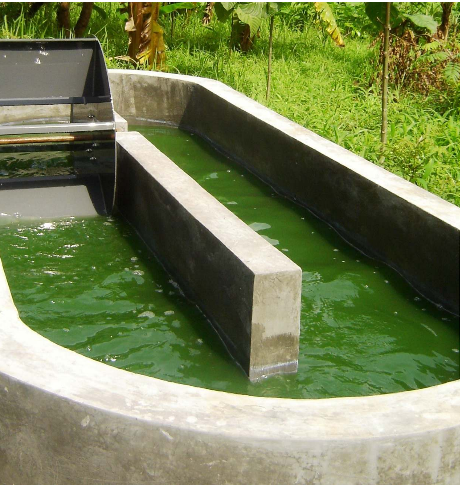
Waste Water Treatment, Universitas Diponegoro
