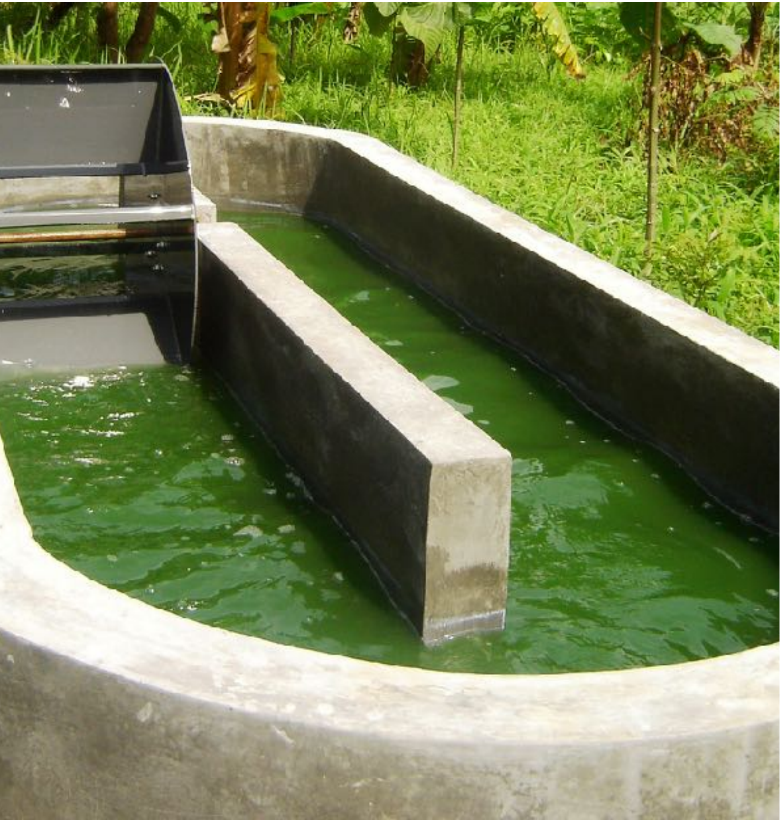
Waste Water Treatment, Universitas Diponegoro
